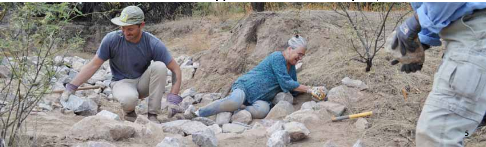
Volunteers build check dams to slow the flow of stormwater and recharge groundwater at Isabella Lee Natural Preserve along the Tanque Verde Creek.
