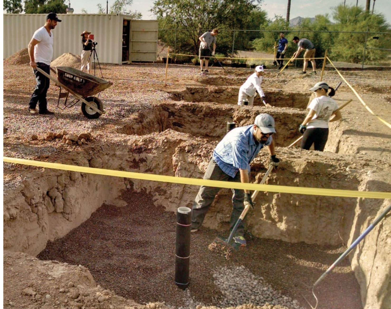
WMG led the installation of experimental water-harvesting basins that will be monitored by ASU and the Flood Control District of Maricopa County. The data collected will help improve green infrastructure design in the Phoenix Valley.
