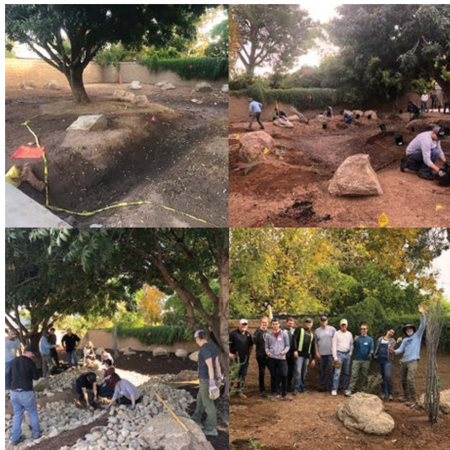
Four Peaks Brewery employees volunteered on a Saturday morning in December to create a public rain garden. They helped shape the basins and berms, armor spillways that collect stormwater off the street, and plant native pollinator shrubs and wildflowers.
